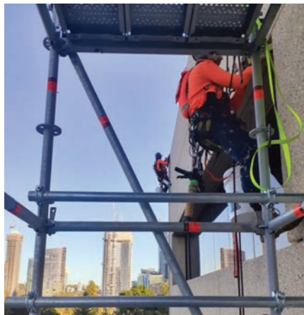
Removing and replacing expansions joints
