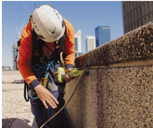
Removing and replacing expansions joints
